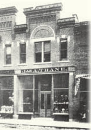
Trane Storefront La Crosse, Wisconsin 1891
